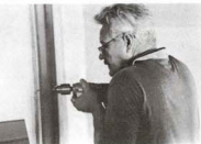
Max Hildman, Oklahoma City, works to transform Quartz Mountain into an arts camp.
